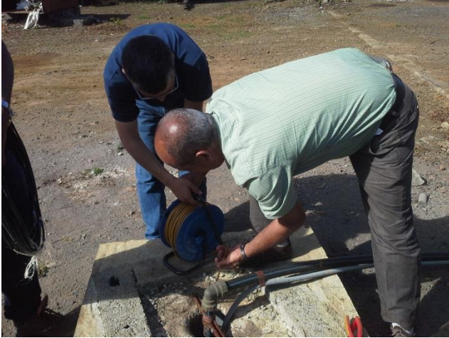
Lowering of probe in the board hole
