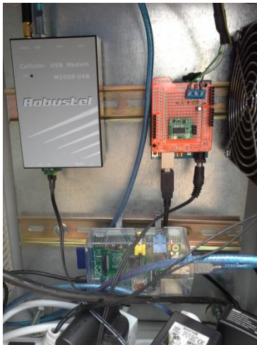
Device electronics mounted inside enclosure
