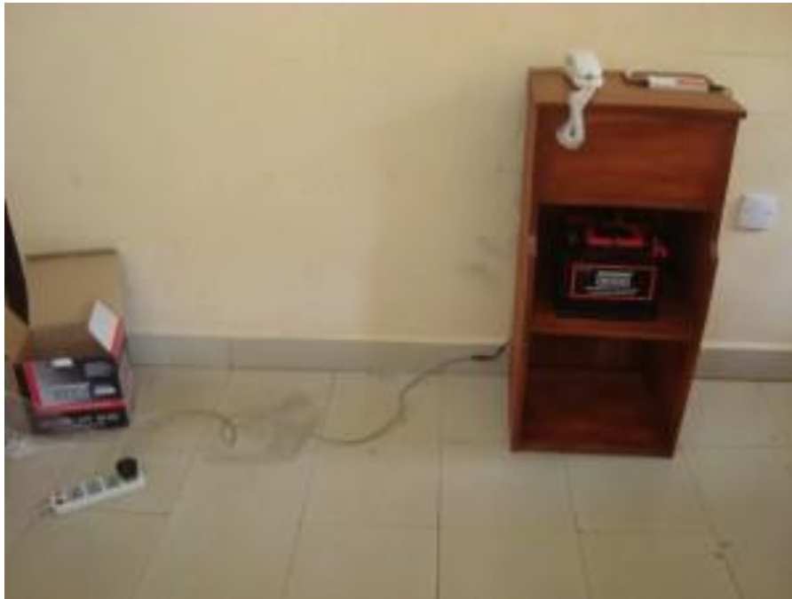
Figure 20: Showing complete set of MP and battery backup
